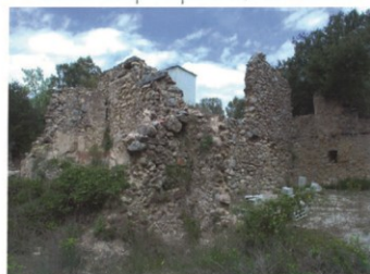
Photo 8. Bât principal . Façade sud
