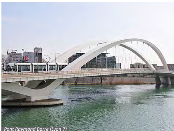
Pont Raymond Barre (Lyon 7)
