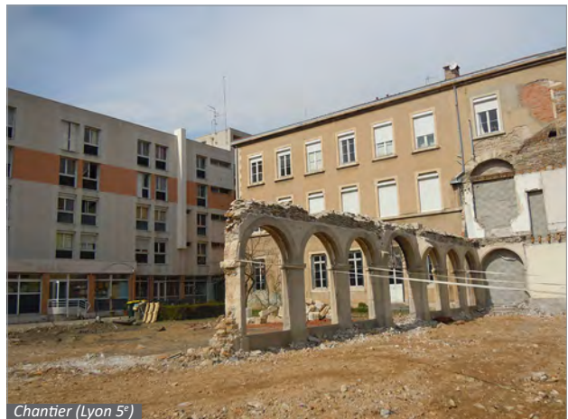
Chantier (Lyon 5 e )
