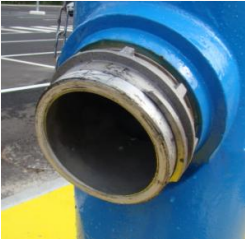
Demi-raccord orientable (sans tenon)
