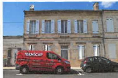
Premier logis, façade principale. Phot. Florian Grollmund IVR72_20143305015NUC2A
