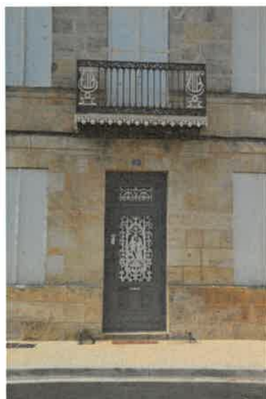
Second logis, travée centrale. Phot. Florian Grollmund IVR72_20143305017NUC2A
