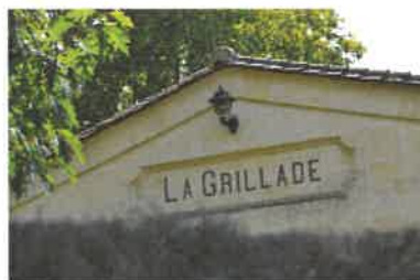
Pignon, cartouche. Phot. Florian Grollimund IVR72_20143306774NUC2A
