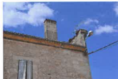
Mur-écran. Phot. Florian Grollimund IVR72_20143304924NUC2A
