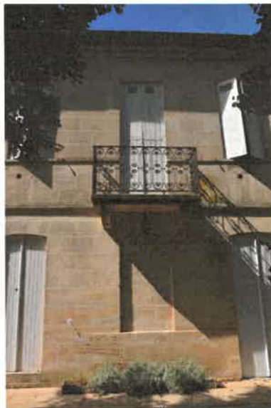
Logis, façade principale. Phot. Florian Grollimund IVR72_20143306181NUC2A
