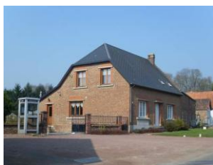
Percements trop larges
