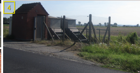
Station de relevage
