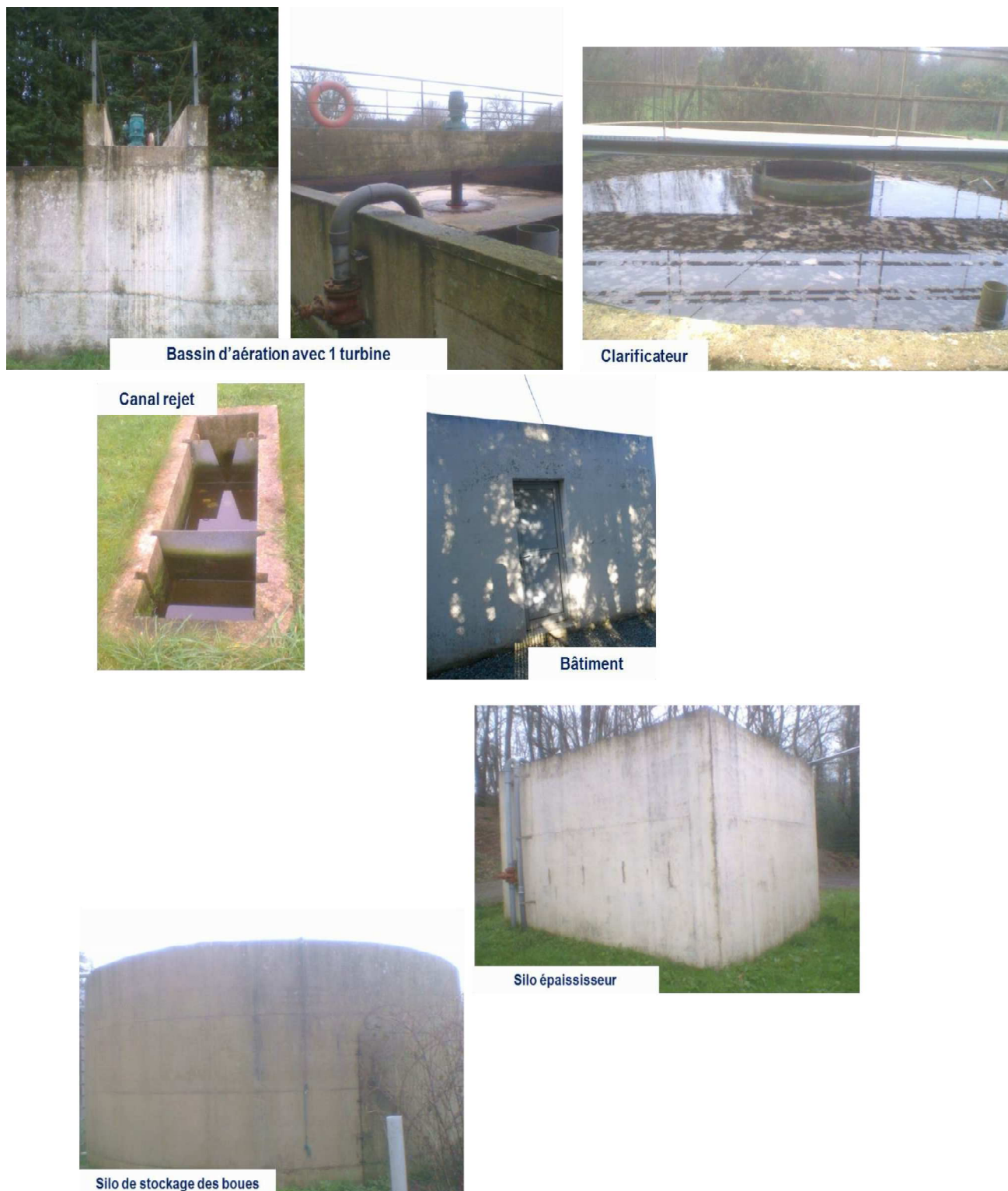
Fig. 17. PRESENTATION DE LA STATION D'EPURATION
