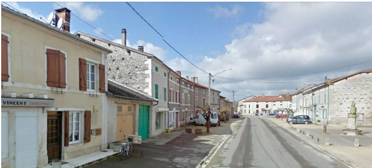
Demange-Baudignécourt – Village de Demange-aux-Eaux
