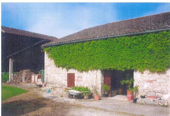
HABITATION EXISTANTE AUX ABORDS DIRECTS
