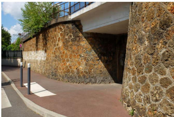
Avenue Fourchon, passage n2
