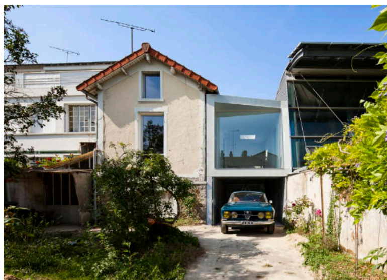
CUT Architectes, extension, Chaville (92) - 2010-2011 © David Foessel & Luc Boegly
