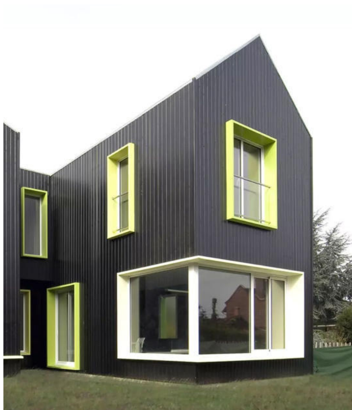
rh+architecture, maison neuve, Clamart (92) - 2009 © rh+architecture
