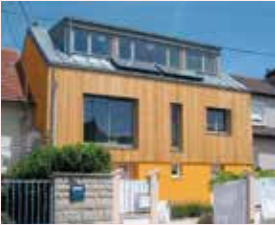
Normier+Postec Maison coque Bagneux © agence Normier + Postec
