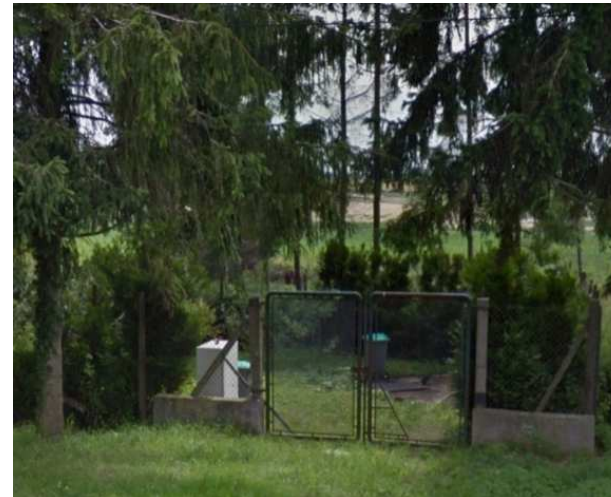
Station de relevage D60, Reinange
